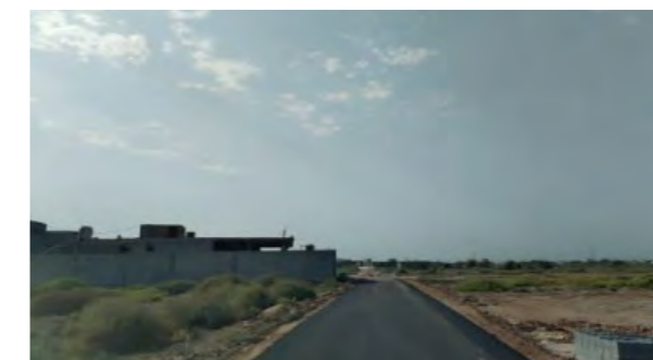
Construction Of General Roads in al Nashwa
