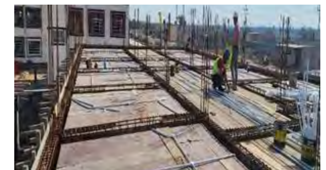
Construction of Al Zuraiji Health Center
